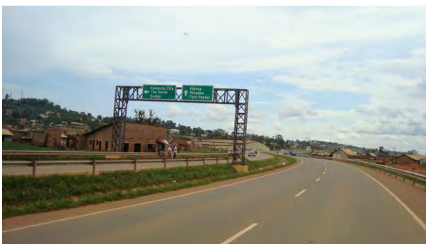
Figure 6-26: Sections of the Northern Bypass/express way. The 1972 design was however altered at implementation. Some sections like this one (right) on the way to Naalya are single carriageways but given the span of the bridges, there is possibility of expanding to dual carriage highways. (Source: Author, March 2010)
