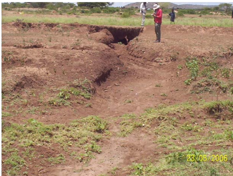
Picture 1: Consequences of lack of maintenance of a soil bunding
