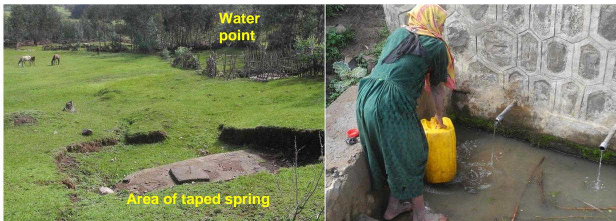
**Photo 21: Very small protection zone around the water point (background), no protection around the taped spring (foreground); whole area used for grazing with problem of contamination**
